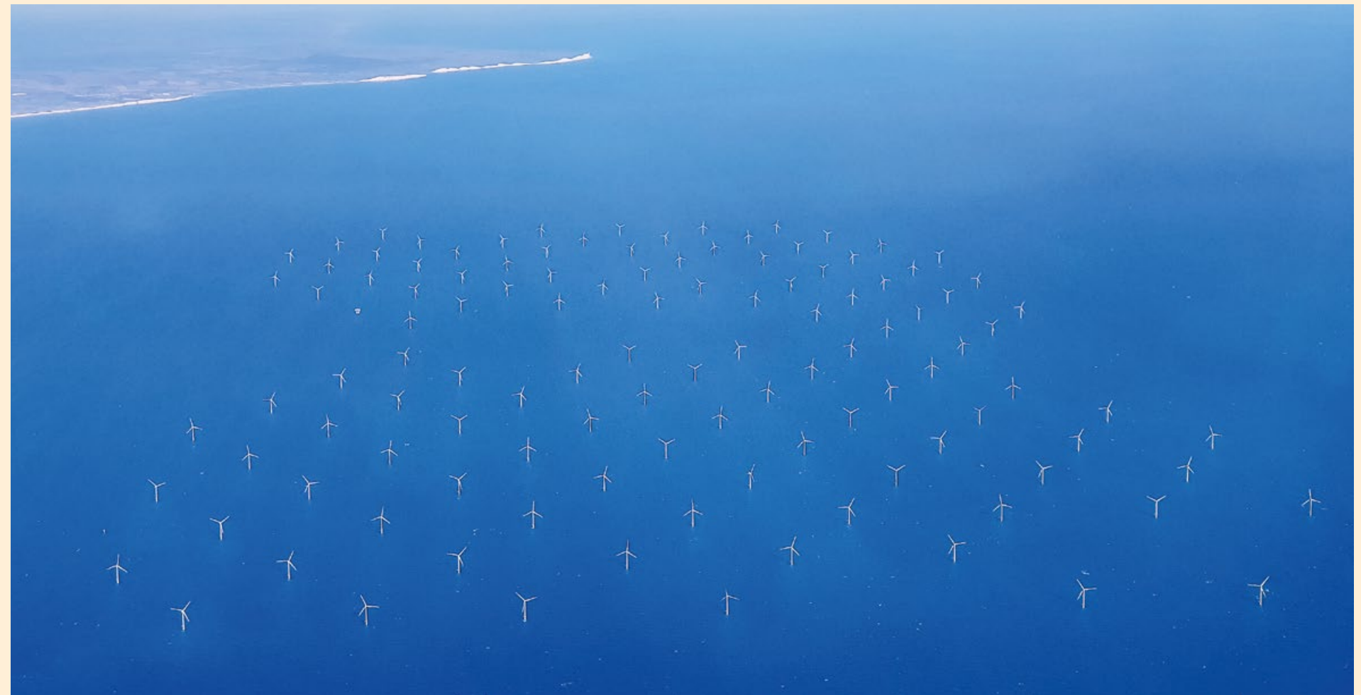
→ Aerial view of the Rampion wind farm which has a total of 116 turbines that power the equivalent of 350,000 homes.
